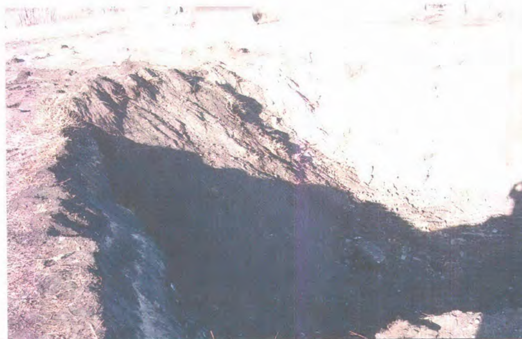
6) Looking northwest. Beginning backfill activities.
