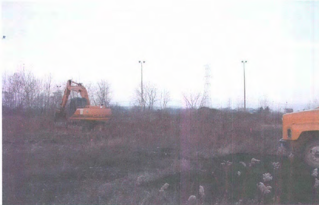
1) Looking west. Before excavating.
