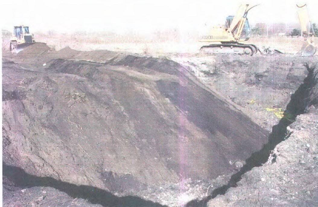
8) Looking north. Backfilling.
