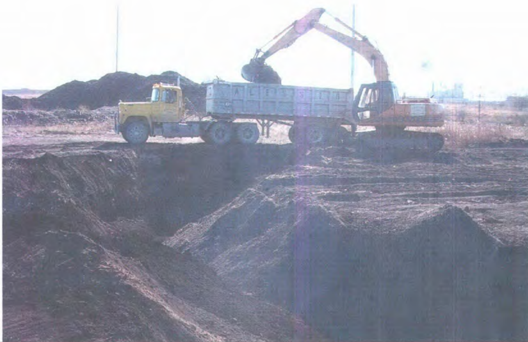
9) Looking south. Loading last load at south end of excavation.
