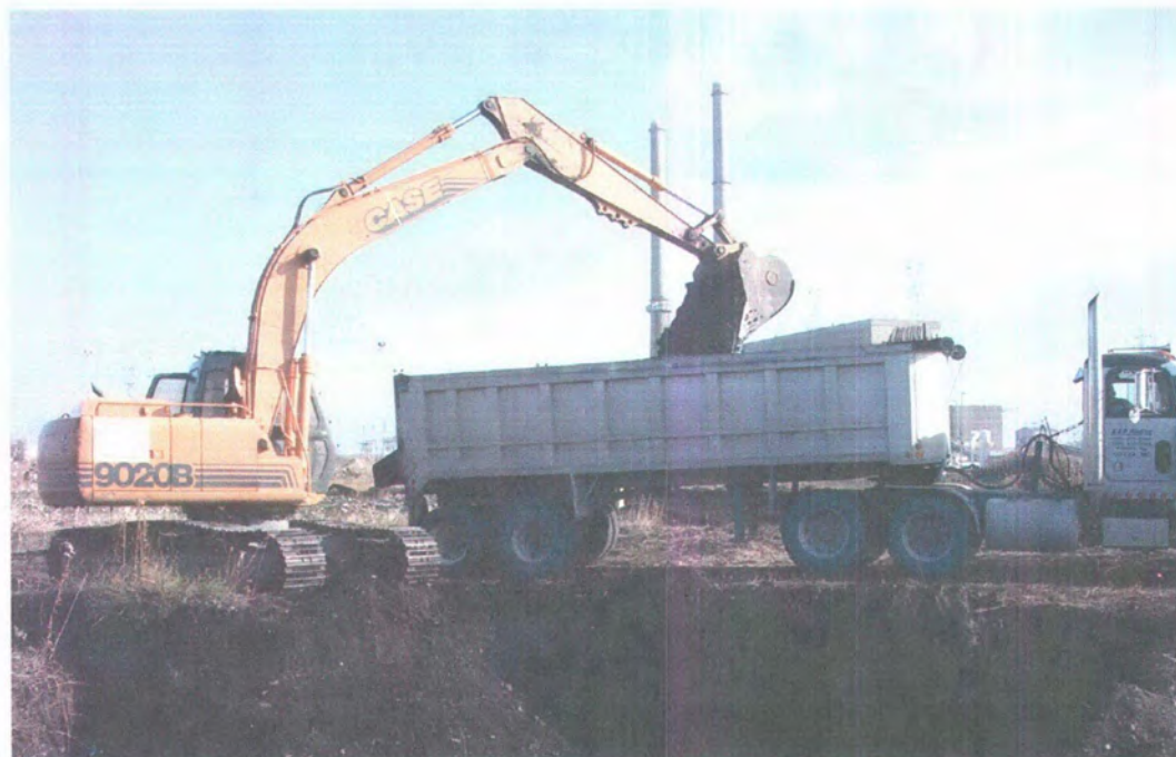
2) Looking east. Excavator loading haul truck.
