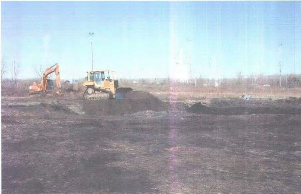
7) Looking north. Backfilling activities.
