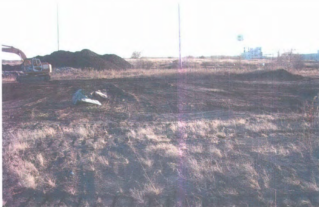
10) Looking south. Completed backfilling.
